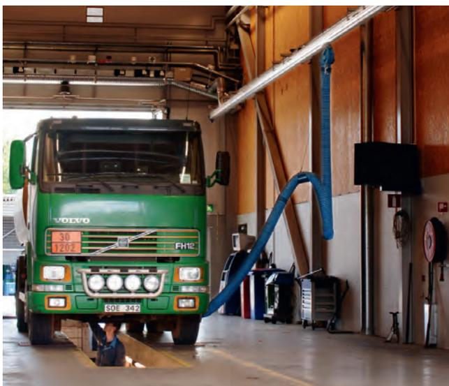
Example exhaust system for vehicle inspection.
