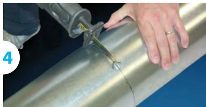
4 Cut off pipe. Saw off pipe.
