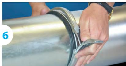
6 Lock the QF strap over the rubber ring and one end of the covering pipe.
