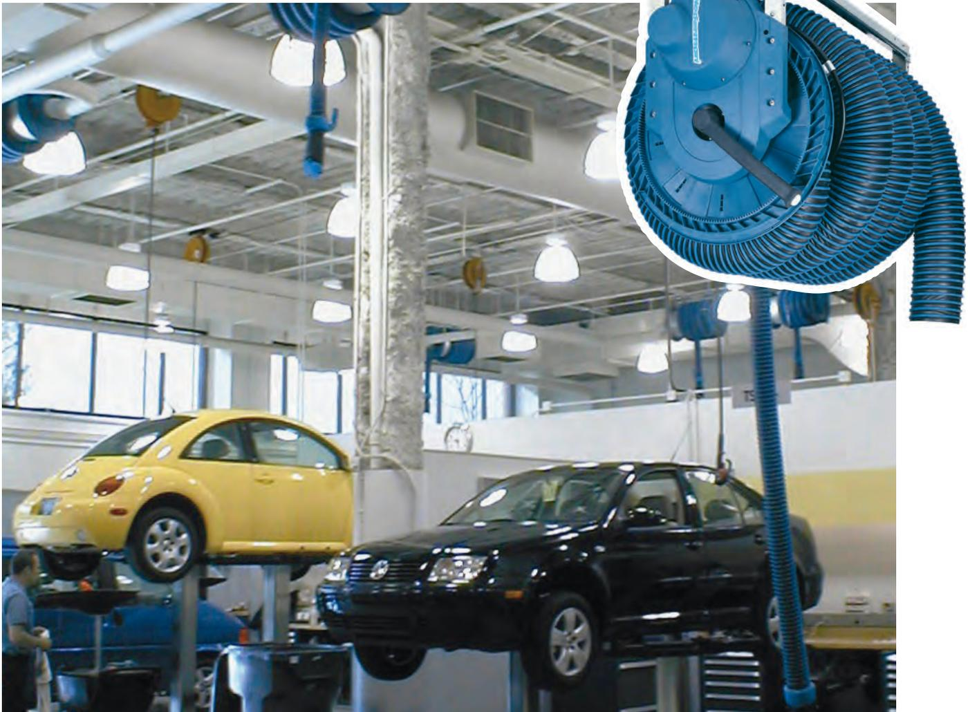
The best solution in workshops with a high ceiling, where overhead cranes etc. have to be considered, or where high vehicles must pass. Operated via a hand unit either an IR control or pendant control. A receiving eye on the reel shows the status of operation. Electronic limit switches reduce the risk of malfunction and unnecessary wear on the hose. Fan start/stop is automatically controlled. Mounting of fan on reel is possible.
